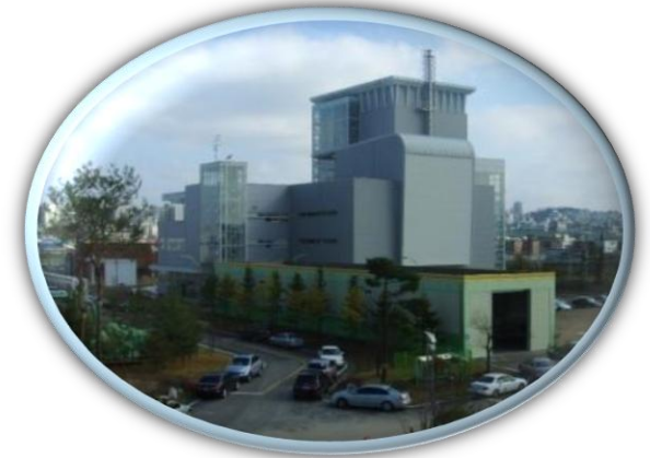
Sewage Sludge-to-Fuel Plant
