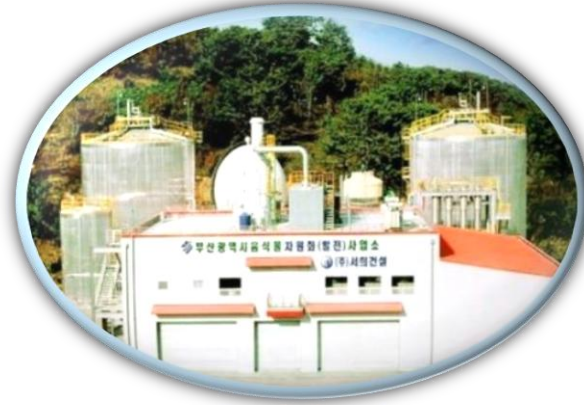
Food Waste-to-Biogas Plant, Busan
